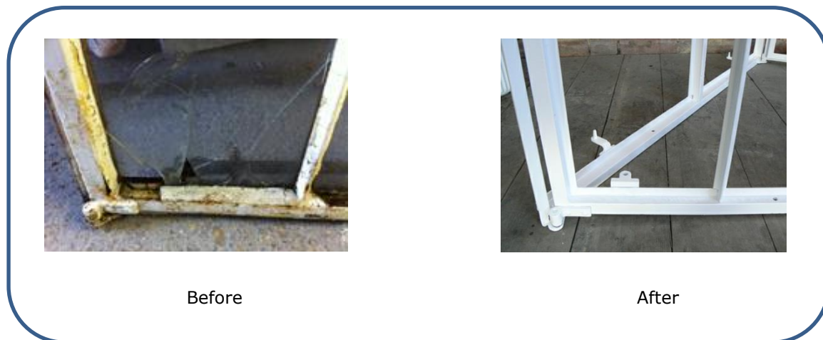
Fig 6 Example of metal repair
