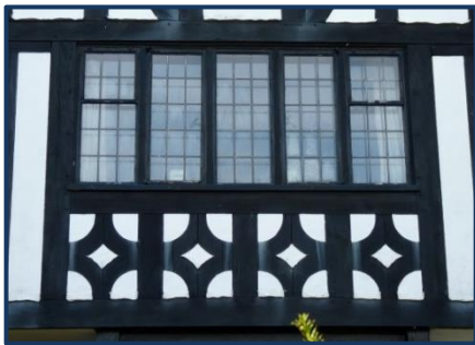
Left: Top hung hinged casements with centrally located fixed lights Right: Side hung hinged casements with centrally located fixed lights
