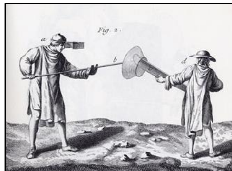
The globe is opened out at one end to form a bowl
